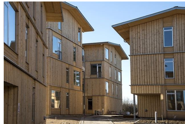
Vandkunsten Architects, DK, Use of timber post-beam and CLT (hybrid construction): Design for disassembly/deconstruction.
