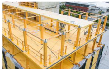
Vandkunsten Architects, DK, Use of timber post-beam and CLT (hybrid construction): Design for disassembly/deconstruction.
