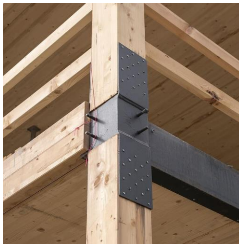
Vandkunsten Architects, DK, Use of timber post-beam and CLT (hybrid construction): Design for disassembly/deconstruction.
